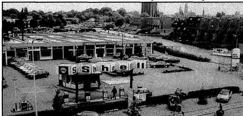
LPG station Friese straatweg in Groningen
